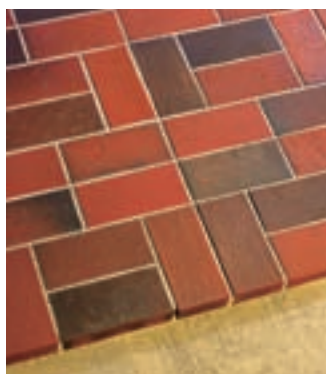
Basket-Weave-Pattern combined with a linear bond. This and similar bonds are less loadable, so they should only be used for terraces etc.
