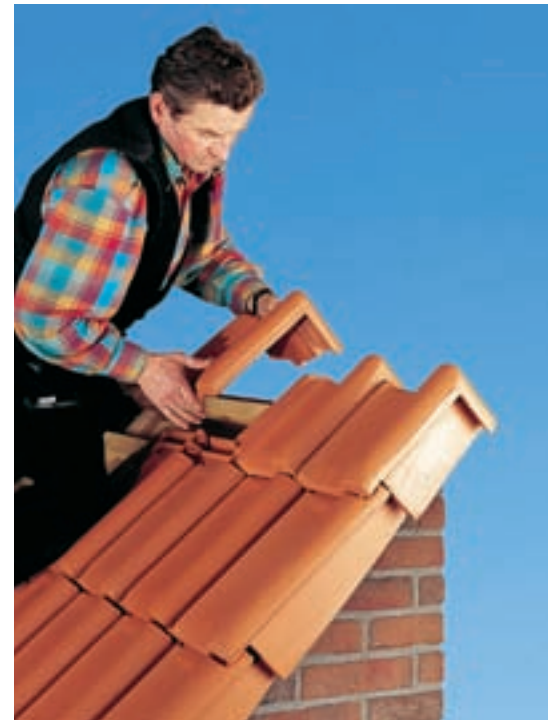
Special verge tiles for single side roofs are developed for the upper end, as well as for the verge that runs along the gable. Roofs with common pitches get a perfect "frame" by using these tiles. Special models for extraordinary pitches are also possible upon request.
