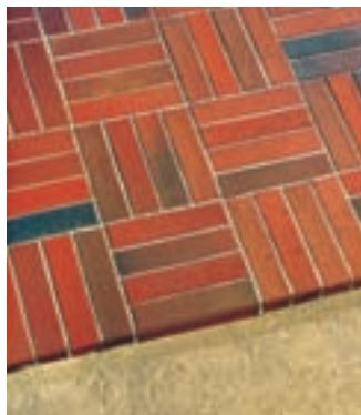
Bundles of four paving bars laid in alternating direction.
