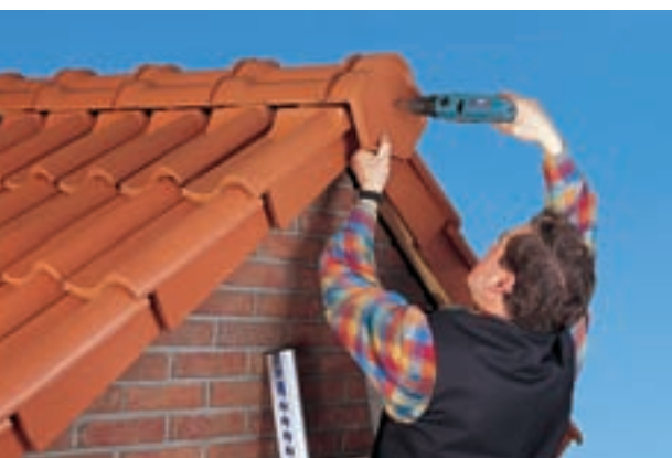
The ridge ends are finished with decorative plates.
